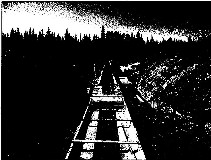
PHOTO 22 – South Embankment Concrete Encasement preparation.
