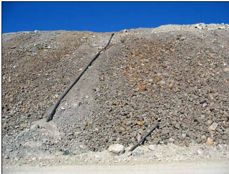
PHOTO 4 – Main Embankment Seepage Collection Pond Return Pipe
