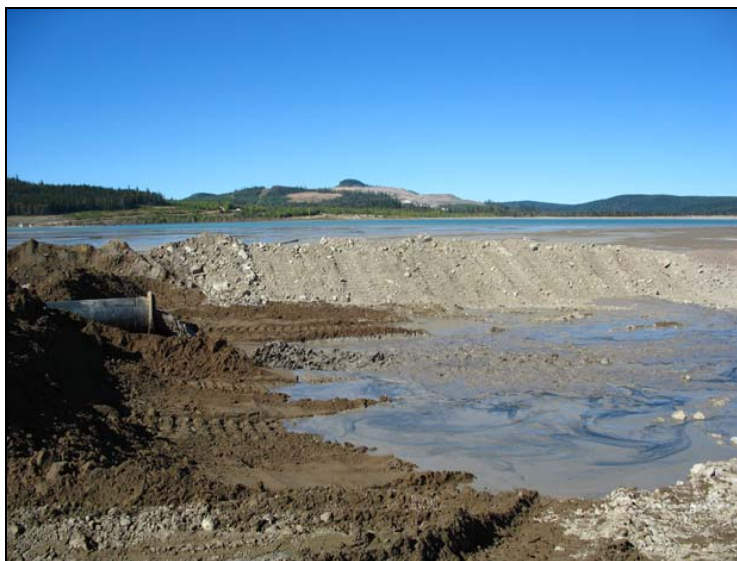
PHOTO 8 – Sand cell construction on Main Embankment.
