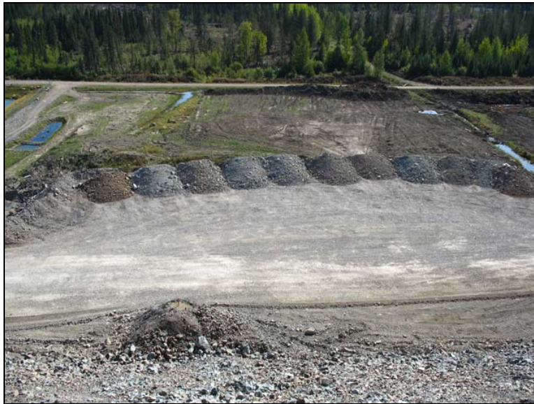
PHOTO 9 – Buttress construction at the Main Embankment.
