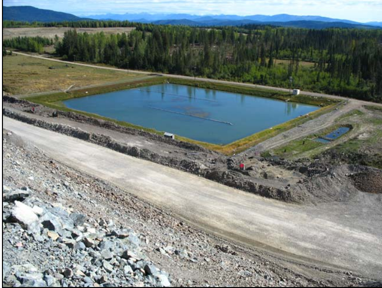
PHOTO 3 – Main Embankment Seepage Collection Pond
