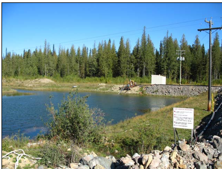
PHOTO 6 – Perimeter Embankment Seepage Collection Pond
