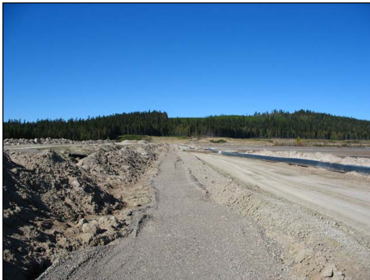
PHOTO 7 – South Embankment upstream toe drain.
