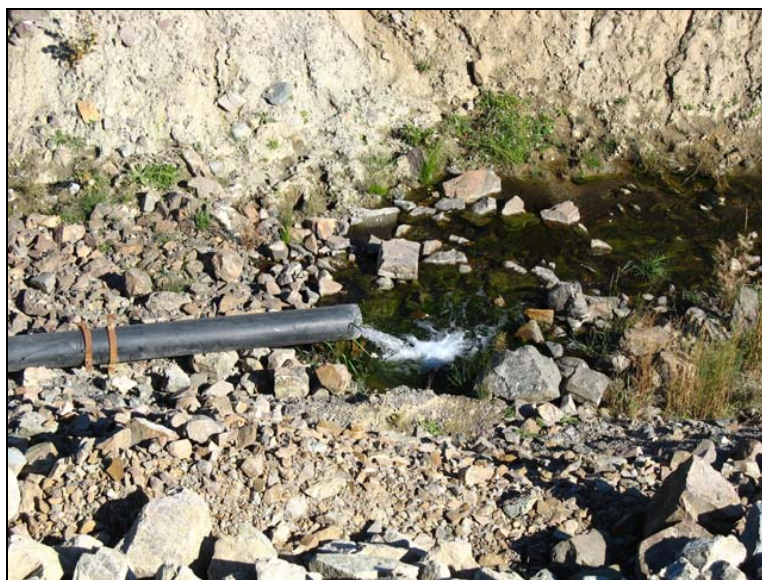
PHOTO 2 – Perimeter Embankment Toe Drain flow.
