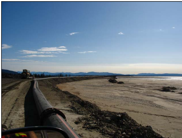
PHOTO 1 – Tailings beach development on the Perimeter Embankment
