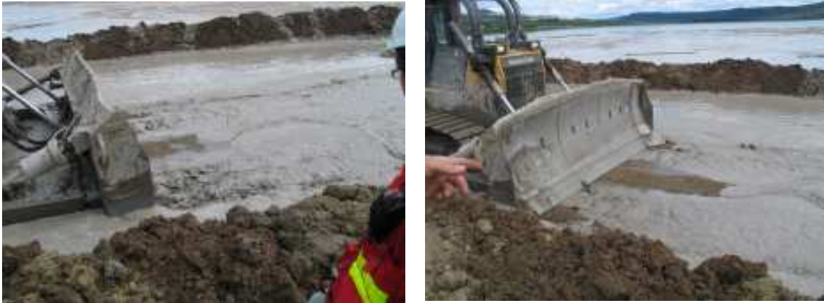
Photo 11 – Cell construction – pushing sand back
