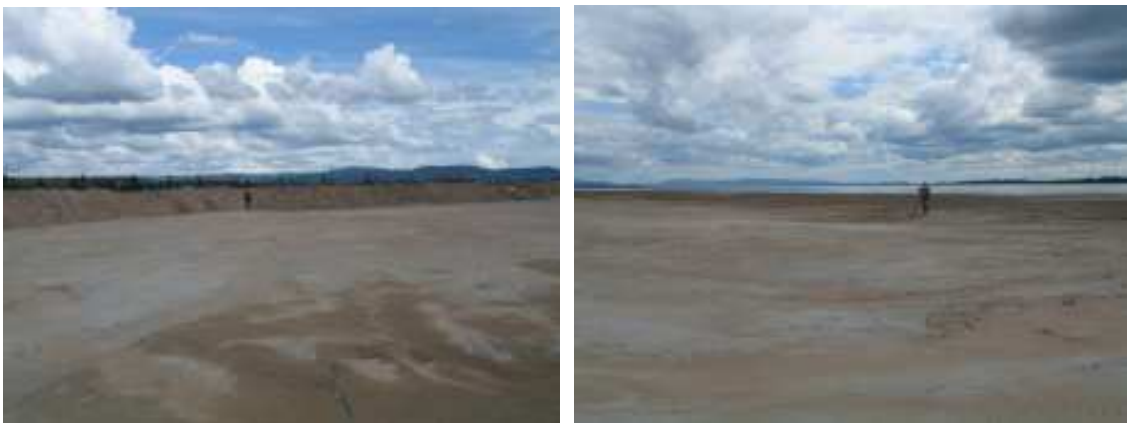
Photo 16 – Typical beach formed by single point discharge of tailings – upstream and downstream view
