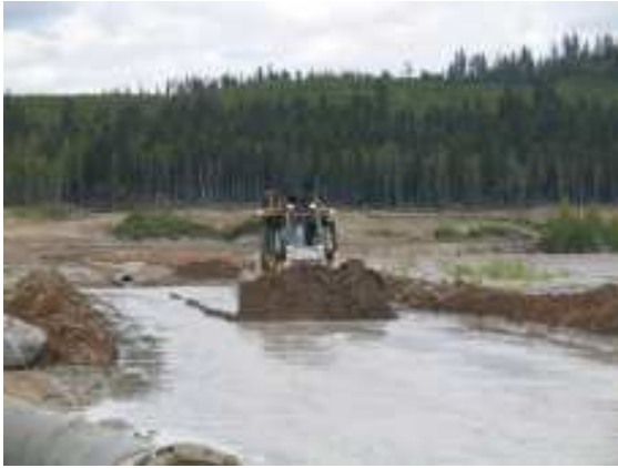
Photo 8 – Cell construction – pushing sand downstream
