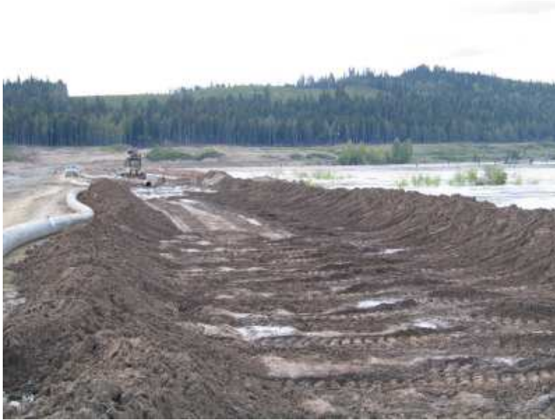
Photo 15 – Bottom of newly prepared cell partially smoothed
