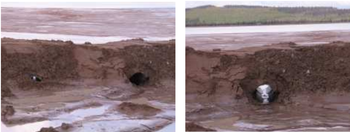
Photo 12 – Re-installed decant pipes
