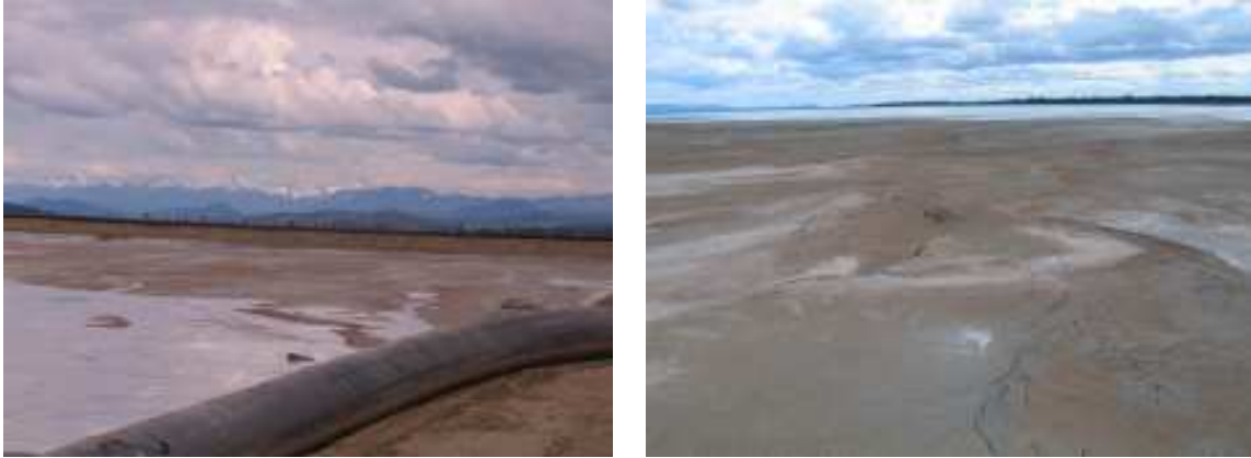
Photo 17 – Typical beach formed by single point discharge of tailings – overview and detail
