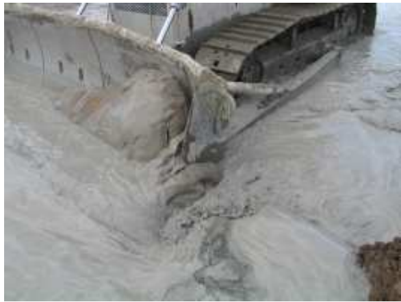
Photo 9 – Cell construction – slimes
