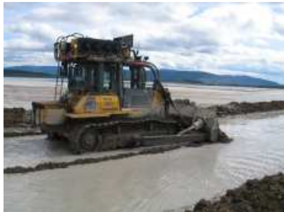
Photo 8 – Cell construction – pushing sand downstream
