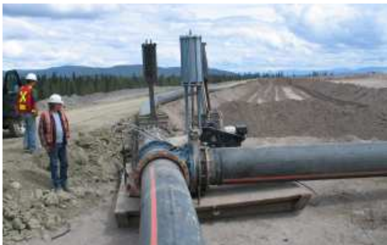
Photo 1 – Preparation for cell construction
