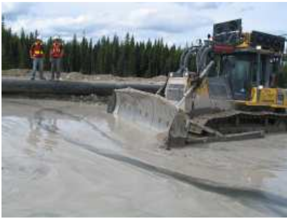
Photo 9 – Cell construction – slimes
