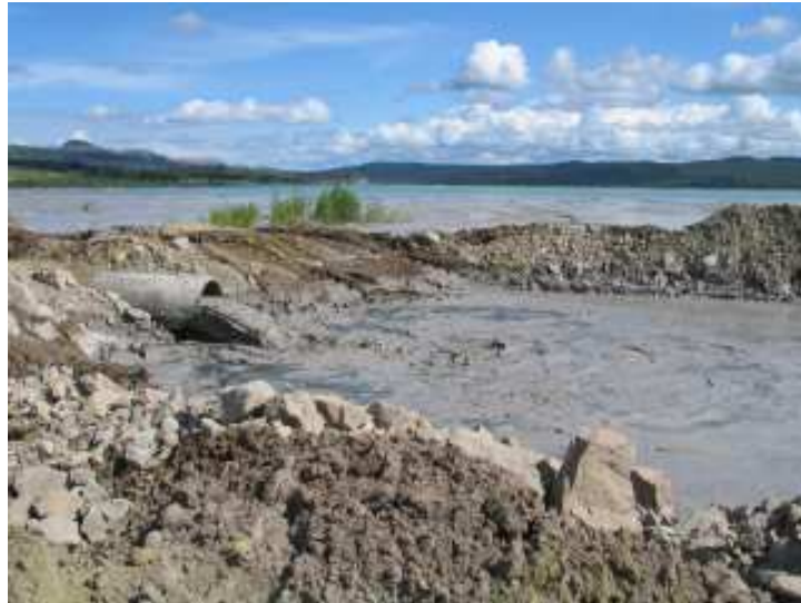
Photo 4 – Flow discharge into the cell
