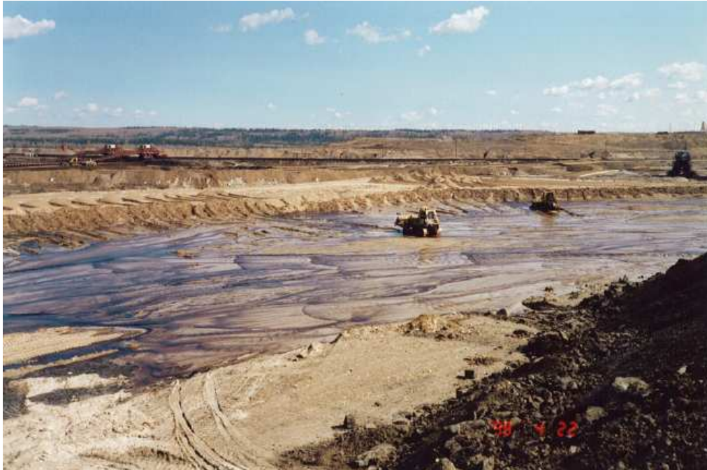
Photo 18 – Dozer operation perpendicular to cell length
