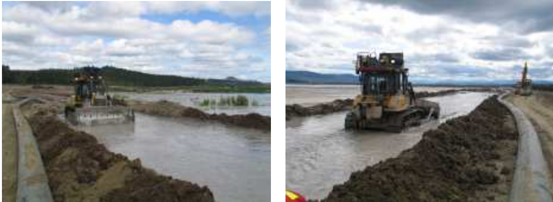
Photo 2 - Cell construction (June 03, 2008)
