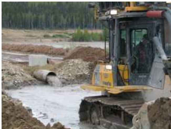
Photo 7 – Cell construction - discharge and dozer
