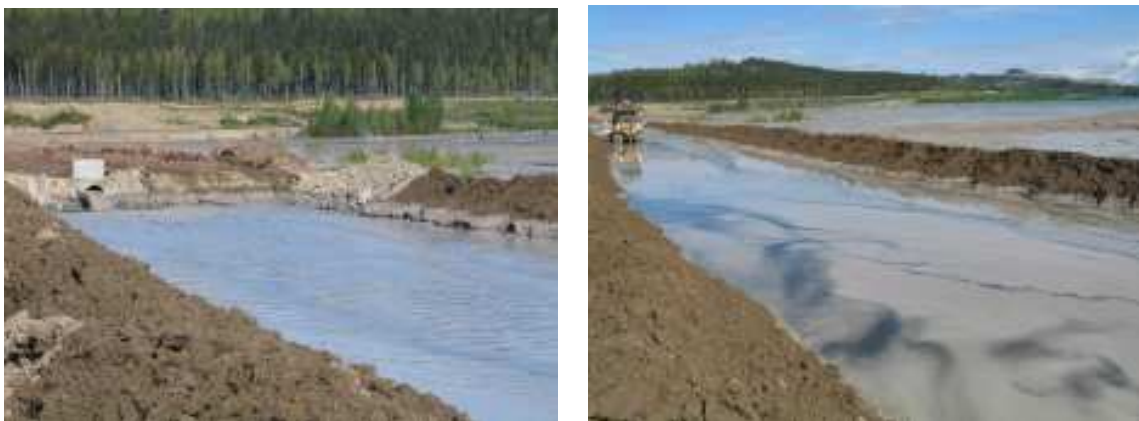
Photo 3 - Cell construction (June 04, 2008)
