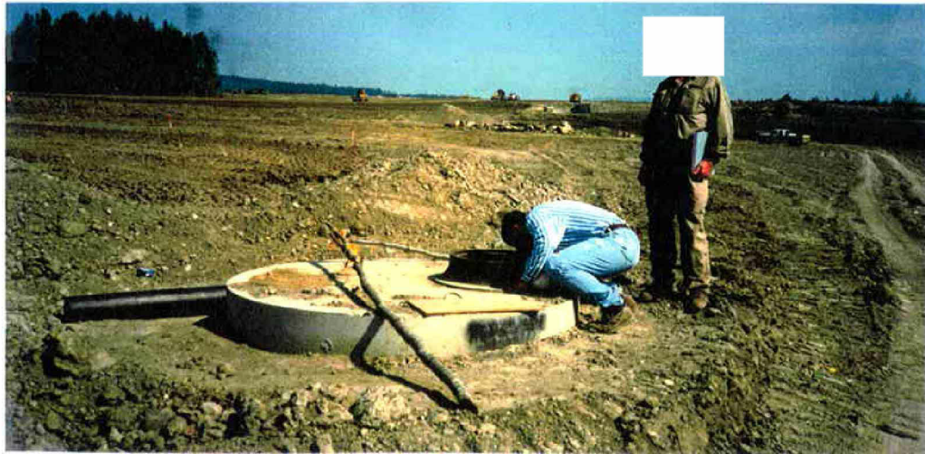
Photo 13. Top of Drain Monitoring Sump at Main Embankment.
