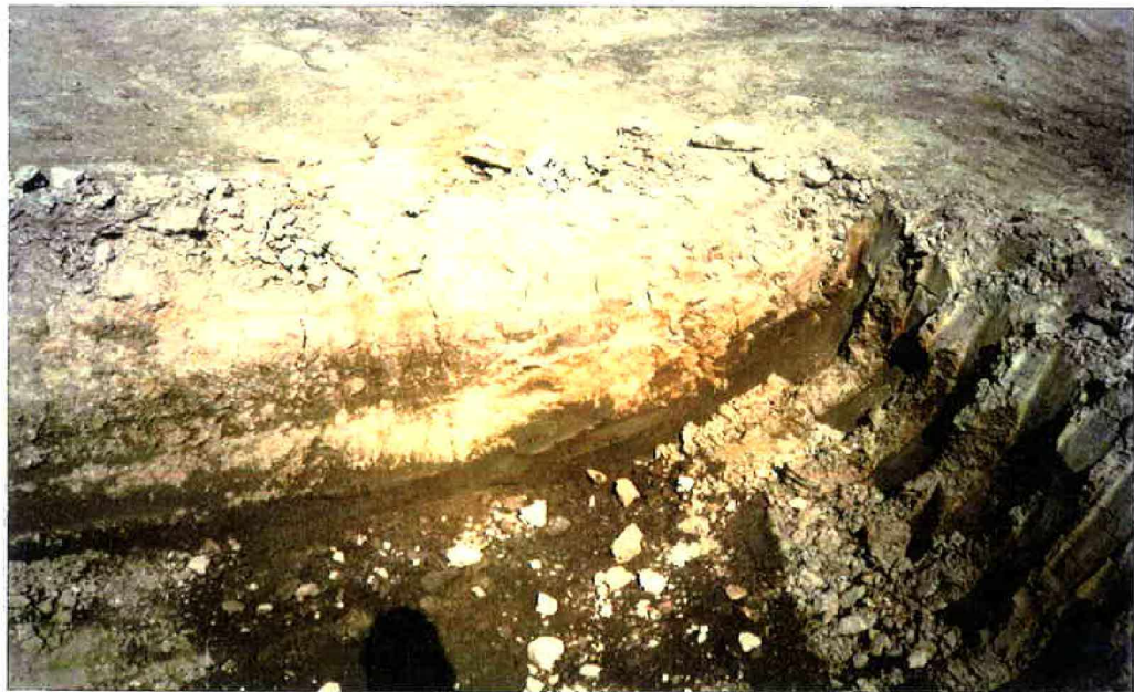
Photo 16. Exploration Trench Near South-West Edge of Basin Liner.
